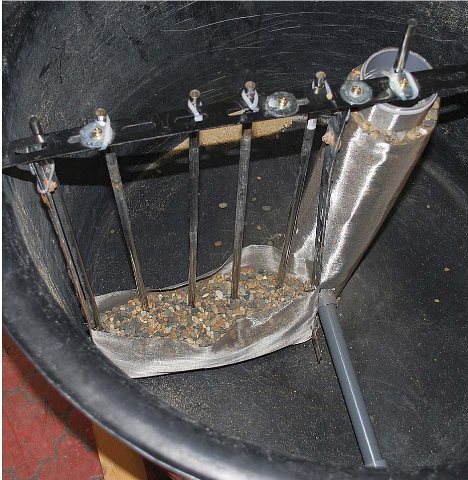
Fig. 3.15: Screened and packed water level tubes and center pipe installed in the tank
