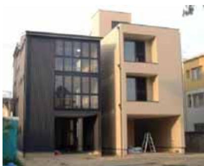
Fig.1 Real wooden frame building
