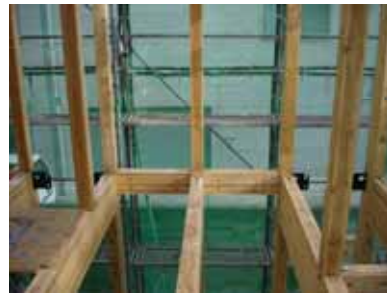
(b) beam removed
