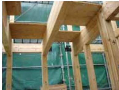
(a) beam removed
