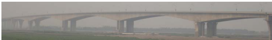
Fig. 1: The figure of Dongying Yellow River Bridge.
